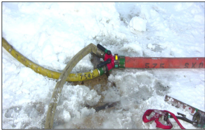
Hooking up another line to a wye may not count as a true back-up line. In the event of supply failure, neither will flow water!
