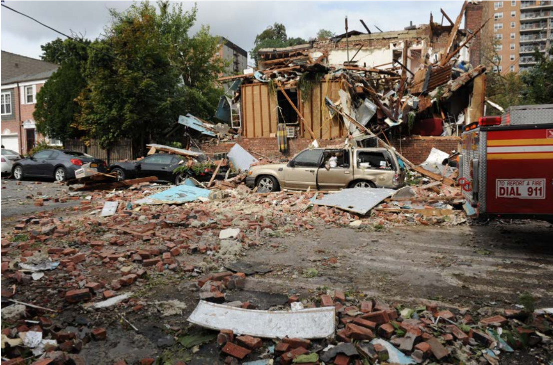
Exposure #2 Post Explosion
