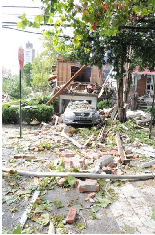
Photo 3 Fire Building After Explosion
